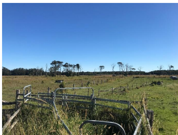
Looking west across the site from the cattle yards towards the earthworks being undertaken on Lot 46
