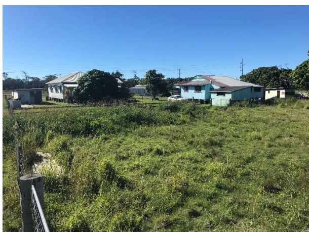
Looking northeast at the two existing dwellings that are located along the northern boundary of Lot 47.
